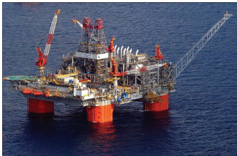
Figure 1. Thunder Horse Platform in the Gulf of Mexico is the largest offshore installation of its kind. Its hull was built by Daewoo Shipbuilding in South Korea, loaded aboard the heavy lift ship MV Blue Marlin , and transported more than 15,000 nautical miles to Ingleside, Texas, where Kiewit Offshore Services integrated the hull with topside modules built in Morgan City, Louisiana. Source: Wikimedia Commons, Andyminicoper.
